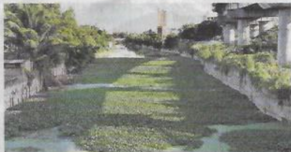
An urban forest will be developed along a 2-km stretch from Madhya Kailash MRTS to Thiruvanmiyur MRTS. •FILE PHOTO
